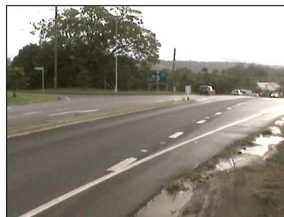
Ewingsdale Rd / William Flick Lane Intersection Looking west
