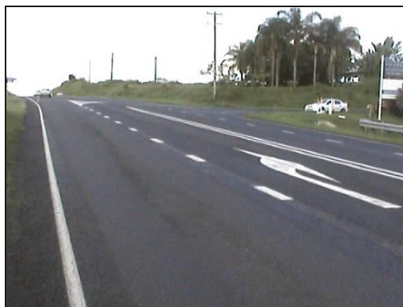
Ewingsdale Rd eastbound approach to McGettigans Lane
